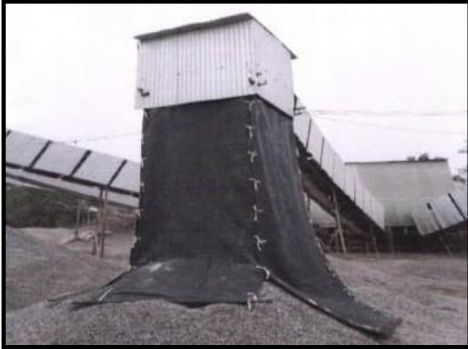
Figure-2: Chute from top of discharge point
