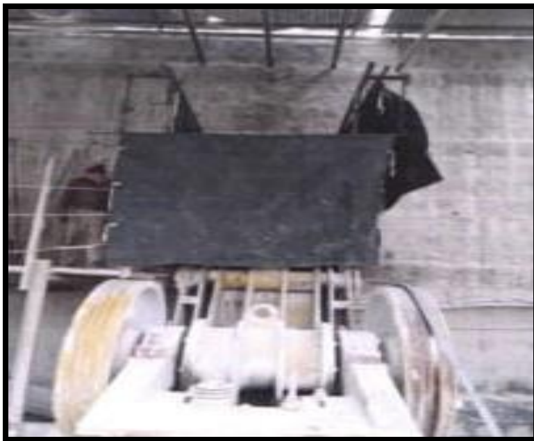
Figure-1: Covering of Primary/Jaw crusher
